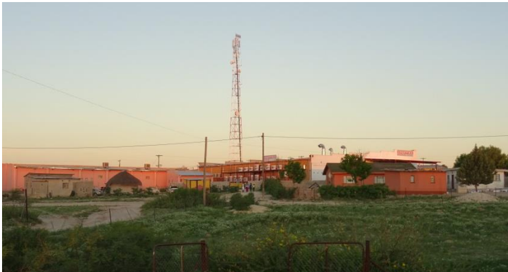
New commercial centre of Letlhakeng, 2016.
