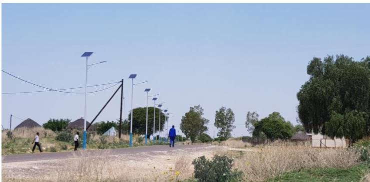
New road lighting, 2017.
